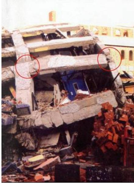
Picture 4. Column-beam connection problems
