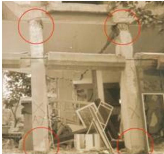
Picture 3. Problems at the points of connection of beam end and a column
