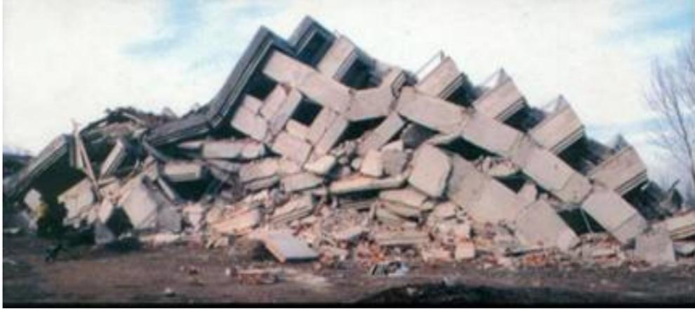
Picture 1. A reinforced concrete framework apartment house collapsed in the earthquake in Kocaeli [12]
