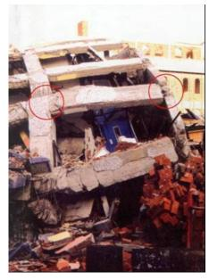
Picture 4. Column-beam connection problems
